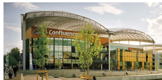
Centre commercial Confluence, Lyon (69)
